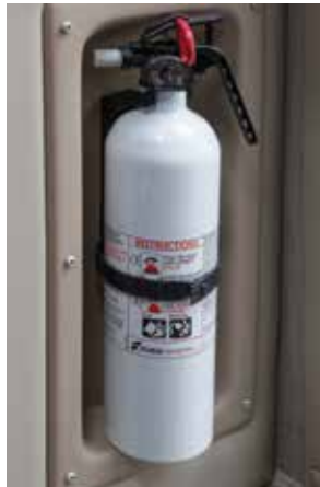
Typical Class B-C fire extinguisher
