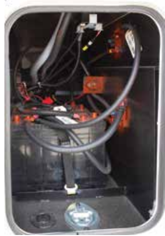
Typical Class A motorhome auxiliary battery compartment
